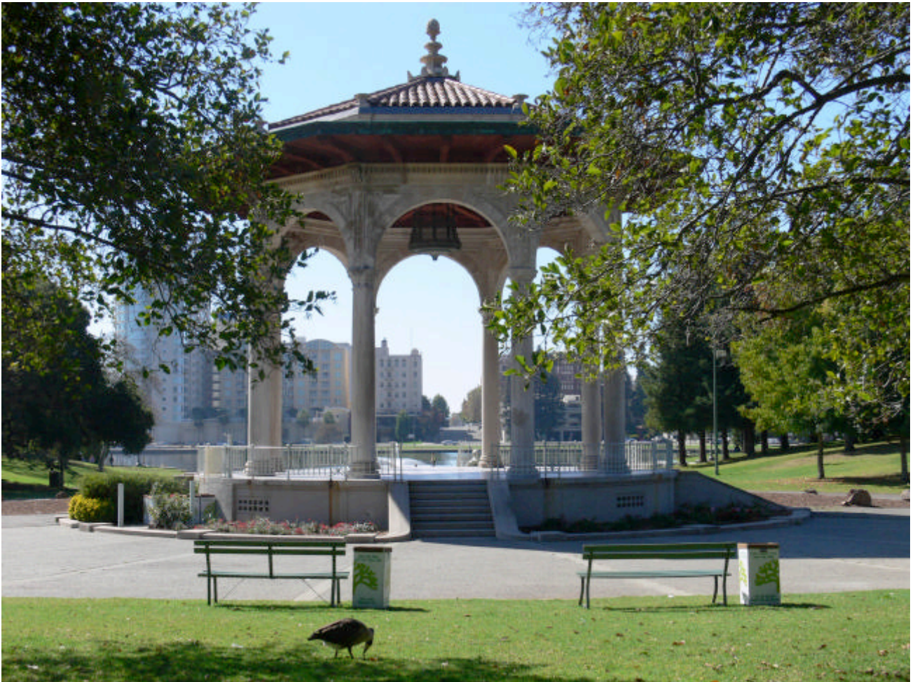
Recent photo shows concrete paving on the North side of the bandstand, and areas of redwood bark that replace former paving on the sides. Historic shrubs have been partially replaced with lower-growing flowers.
