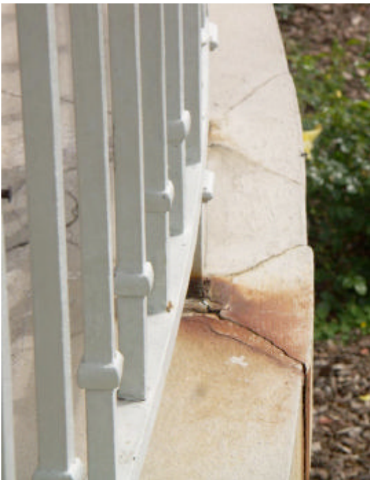
Below: previously repaired spalls about to fail.
