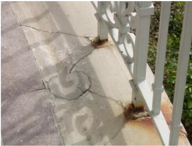
Gutter with filled-in drain at the floor of the bandstand.
