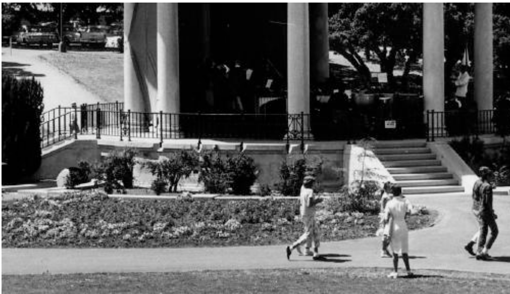
Historic photo from the early 1960's showing planting in the area currently occupied with redwood mulch, and existing black railings. Note also the extensive open spalling at the railing attachments.
