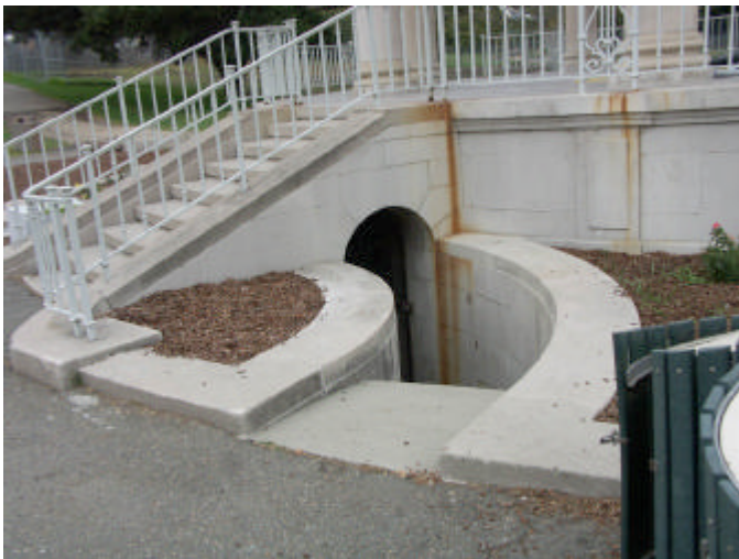
South stair and stairs to basement. Note rust stains on walls.
